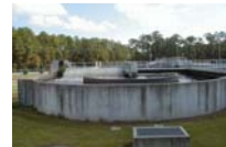
Wastewater treatment facility, Mississippi Courtesy EPA
