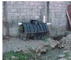
Septic Tank Courtesy EPA
