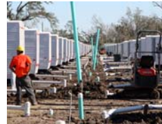
Temporary housing being plumbed, Louisiana Courtesy FEMA
