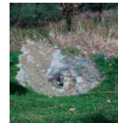
Flooding manhole Courtesy USGS
