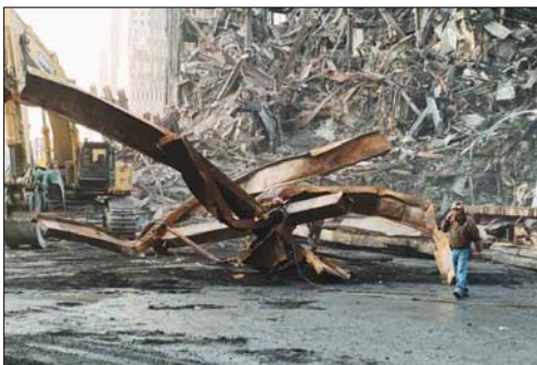
Twisted steel and other debris at World Trade Center site following terrorist attacks of September 11, 2001. Courtesy of OSHA.
