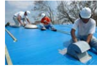
Cutting vent holes for roof, Texas Courtesy FEMA
