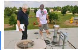
HVAC assessment at a school, Oklahoma Courtesy FEMA
