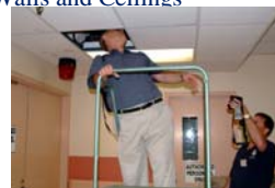
Checking ceiling in a hospital, Hawaii
