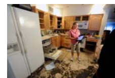
Interior Assessment, Connecticut, Courtesy FEMA
