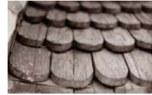
Shingles/roof covering Courtesy National Park Service
