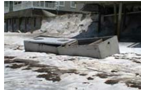
Storm surge removes onsite wastewater system Courtesy CDC
