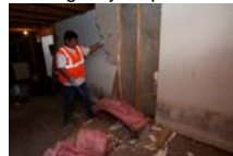
Moldy drywall removal, Montana
