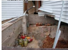
Foundation shifting after tornadoes, Montana
