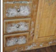
Mold growth on kitchen cabinets, Tennessee
