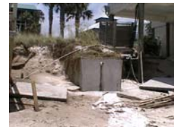
Eroded onsite system, Florida Courtesy CDC
