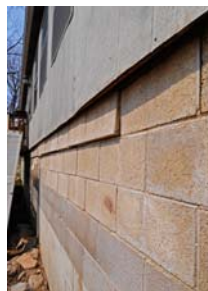
Flood water dislodges foundation, Arkansas Courtesy FEMA
