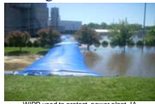
WIPP used to protect power plant, IA Courtesy Hydrological Solutions, Inc.
