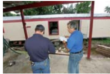
Building assessment, Texas Courtesy FEMA
