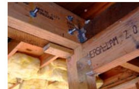
Earthquake straps, California
