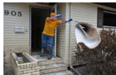
Carpet and padding removal, North Dakota Courtesy FEMA
