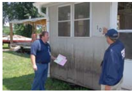
Flooding waterline elevation mark, Montana
