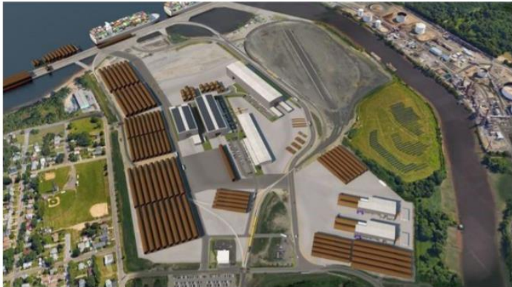
Forthcoming EWW Monopile Manufacturing Facility, Paulsboro, NJ
