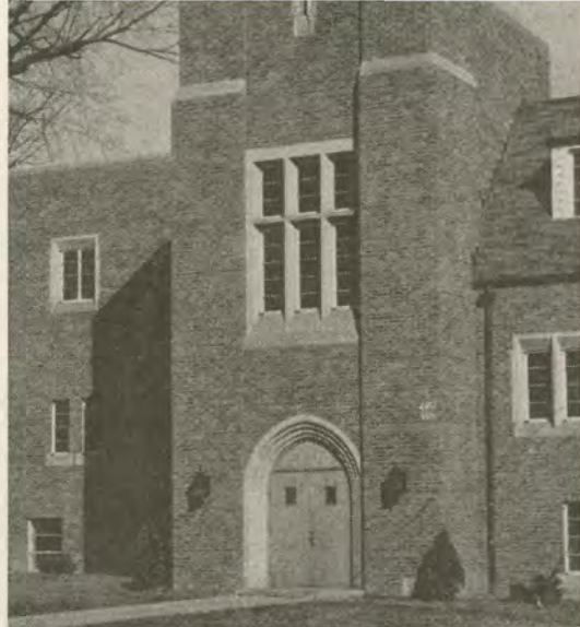
The front entrance to Wesley House.
