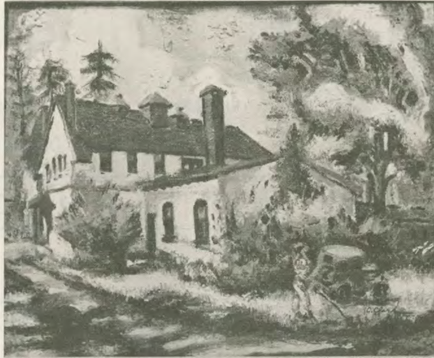
Old Swayne (oldest building on Talladega College campus)
