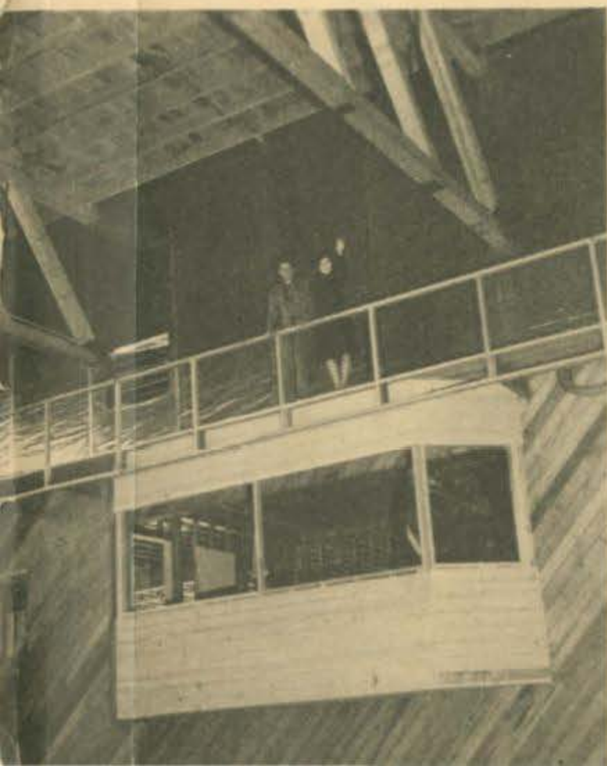
Miss Stefa D'Lys, television production director, and Dave Crandell inspecting the great stage of W6XAO. Note copper sheathing and control room directly beneath
