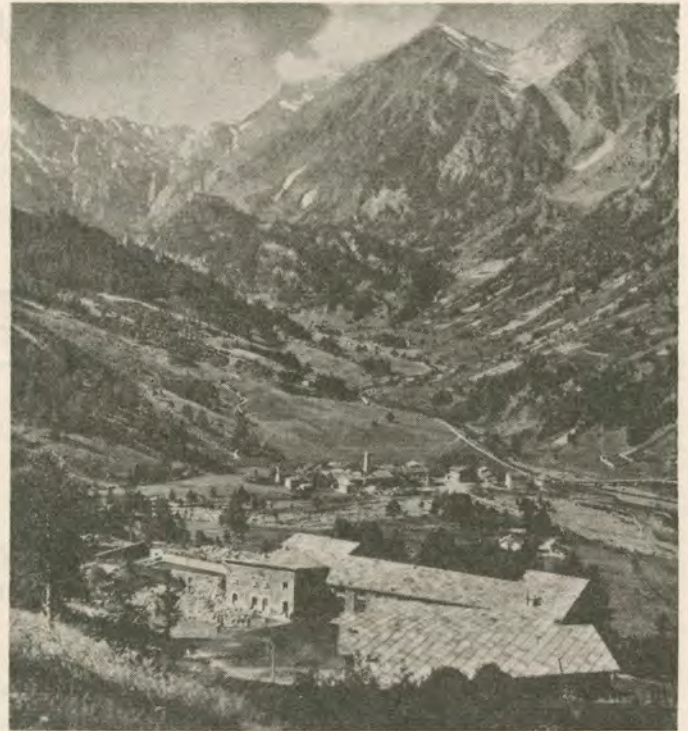
Agape and the Valley of Praly. At the present Agape is formed by four buildings joined by a corridor covering a flight of steps. The buildings consist of one large block and three smaller houses which provide bedrooms for the guests.
