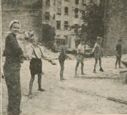
One method of transporting bricks. The receiver is Pat Nelson, wife of the author.
