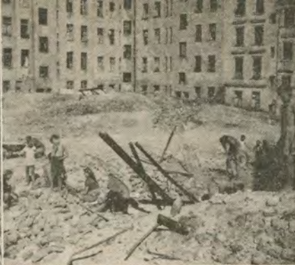
This is how the site looked when the work first began.
