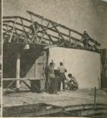
Taking down army barracks for use as neighborhood center.
