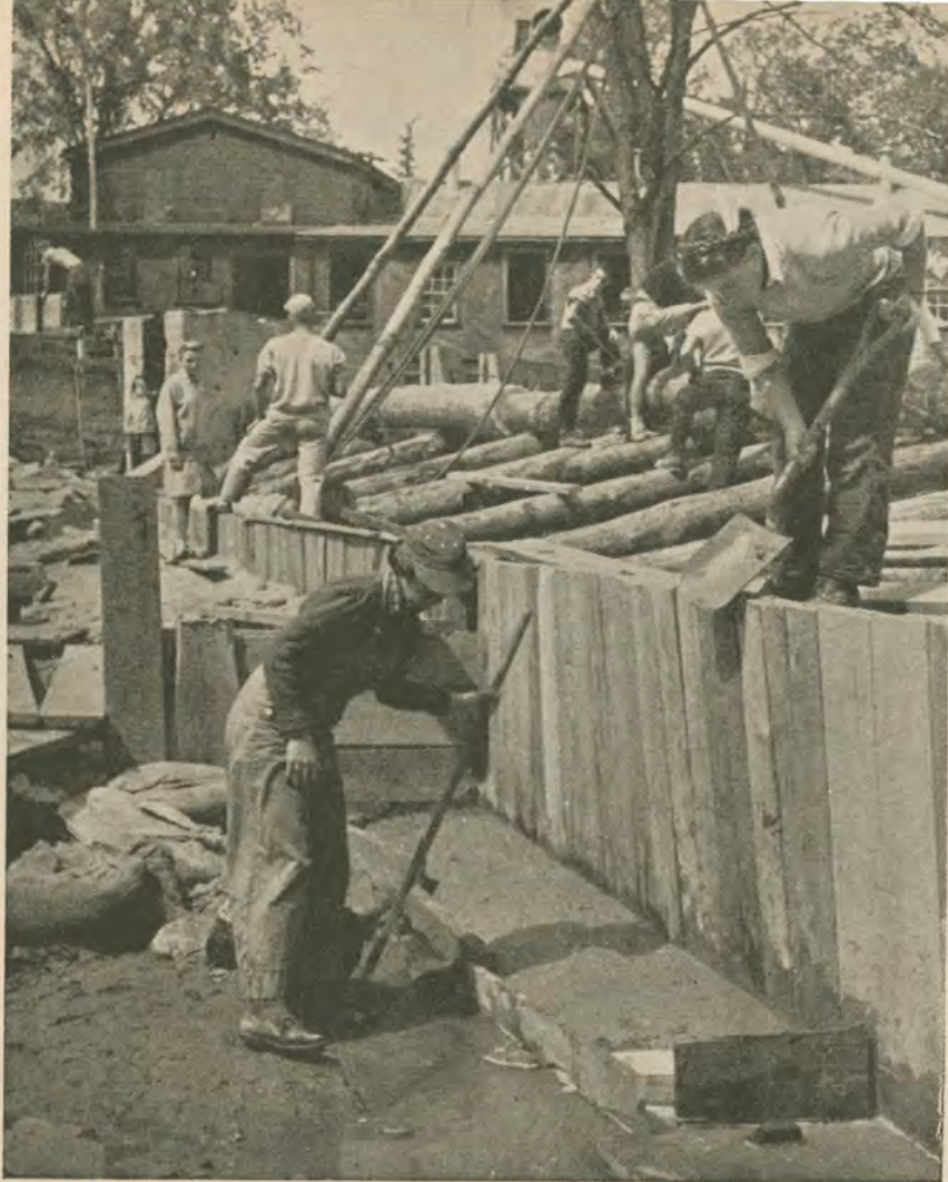
Construction work in this Negro neighborhood in Philadelphia gives this AFSC summer worker a chance to improve racial relationships in this housing area.
