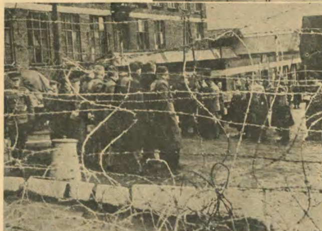
... And always the ugly-looking barbed wire.—Photos courtesy of the WSSF
