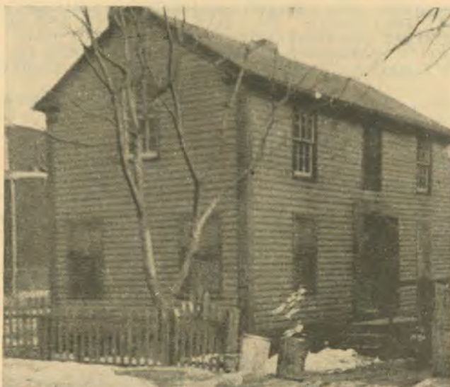
The house at 50 Chadwick Street
