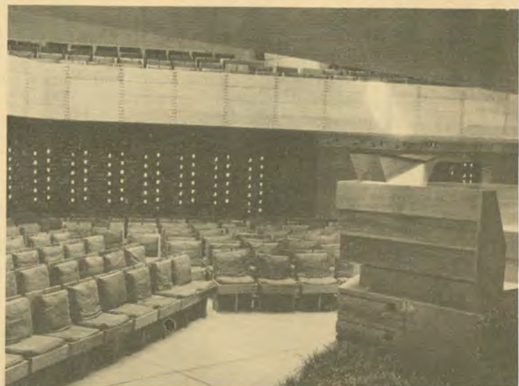
Annie Pfeiffer Chapel. View looking out from platform behind speaker's rostrum. Students worked on the Chapel in shifts, going to classes three days a week and working on three other days, and finished it in a year and a half. It is the first and center building of the E. Stanley Jones Foundation on the campus.
